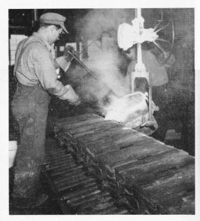
(5) The crucible of molten brass is carried along an overhead track to a row of molds ready for the pour. Robert Whiteway mans the hoist wheel, Ferdinand Nadeau pours metal into molds.
