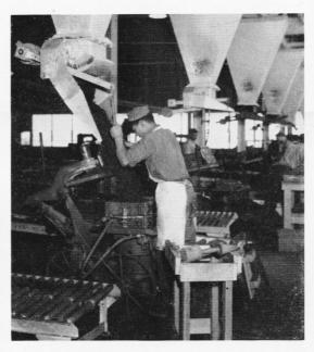
(4) The next step is to pack the flasks. Fred Trotman releases the trip which allows the sand to drop from the conveyor belt into the flask where it is pack down well.
