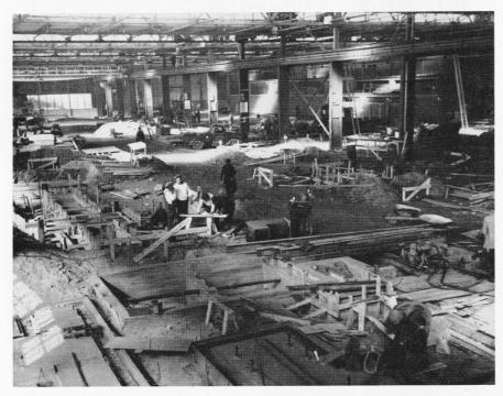
From a position in the south corner and looking north, the ground in the East Mill Addition seems to be torn up in a series of excavations of various sizes and shapes. They are for the foundations of the heavy machinery which will be set up in the New Mill. In the foreground can be seen the anchor bolts in the foundation for a Roll Grinder. In the left background can be seen the foundation for a huge motor generator.
